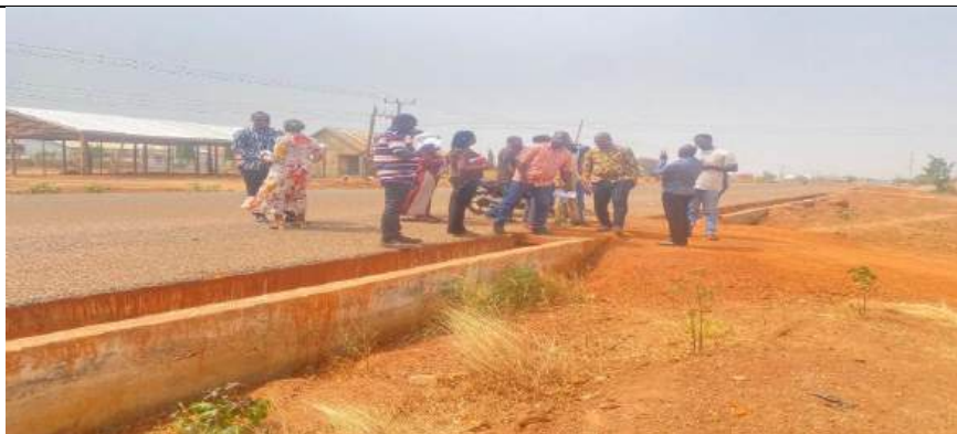
MONITORING OF KPALSI- DIMALA ROAD CONSTRUCTION
