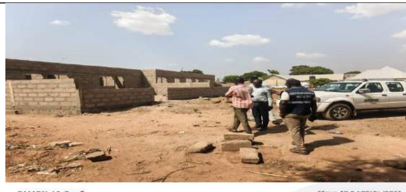
MONITORING OF CHPS COMPOUND CONSTRUCTION AT SOGNAAYILI
