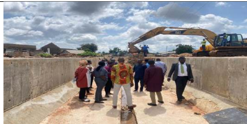
MONITORING OF STORM DRAIN CONSTRUCTION ON THE NALURO- NOBISCO STREAM
