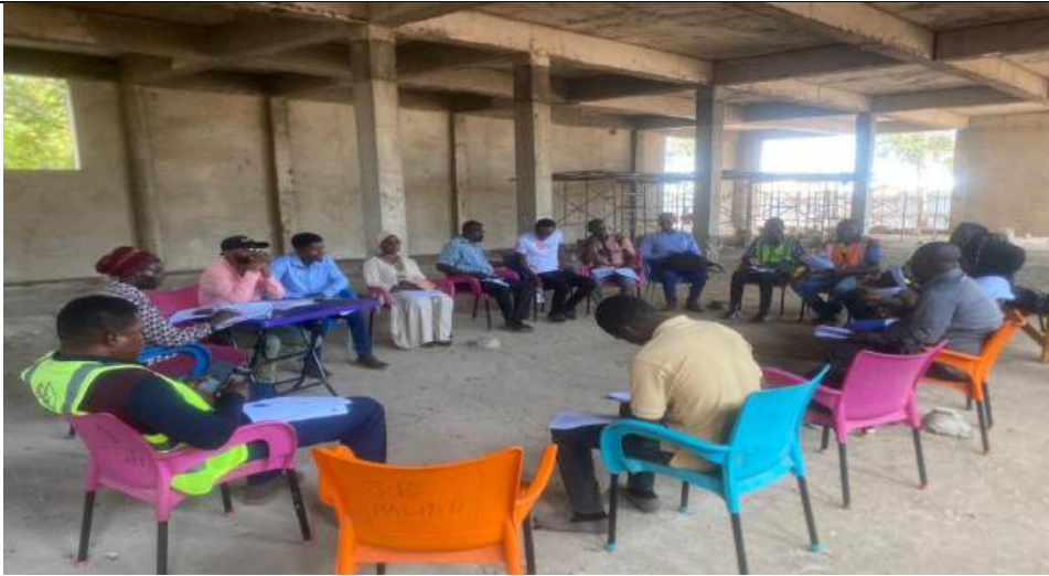
SITE MEETING AT KATARIGA COMMERCIAL BUILDING CONSTRUCTION
