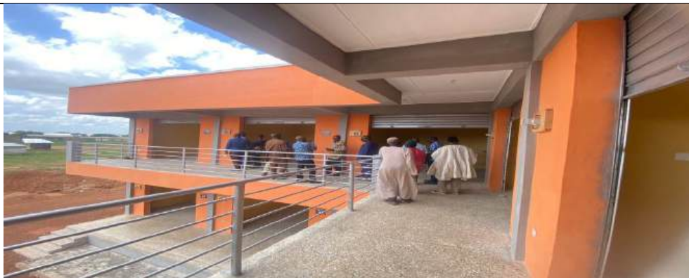
MONITORING OF CONSTRUCTION OF 24NO. MARKET STORES AT SAGNARIGU MARKET
